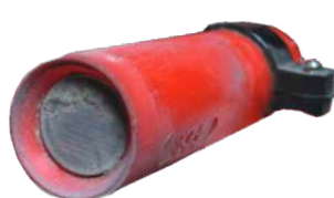
Dirty photocell which can result error in ignition or flame dissappear error
